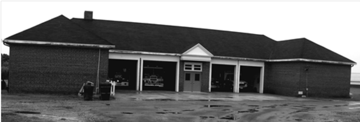
Figure 4: Saxis Firehouse and Town Office – Located in Flood Zones. Photo by Elaine Meil
