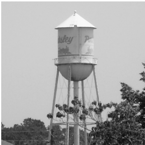
Figure 3: Parksley Water Tower. Photo by Curt Smith
