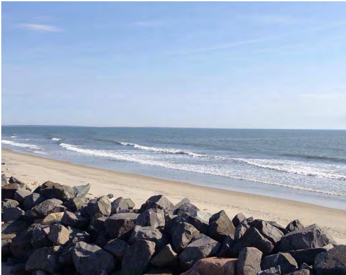
Figure 7: Revetment at the beach of Wallops Flight Facility. Photo Credit: NASA
