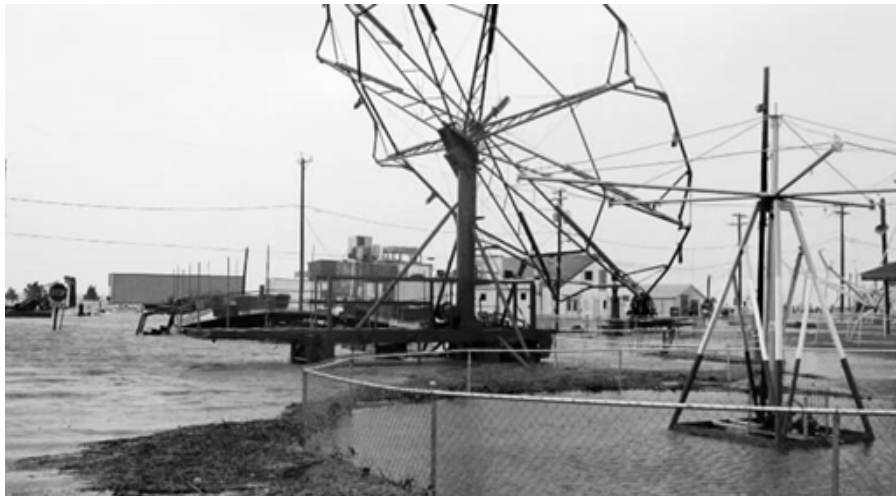
Figure 15: The carnival grounds in Wachapreague are at risk to coastal flooding and were inundated with flood waters from Hurricane Isabel in 2003. High winds and lightning also threaten these structures. Photo by Dan Bilicki
