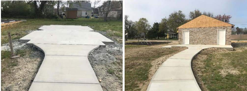
Sidewalk, restroom landing and pavilion slab have been placed.
