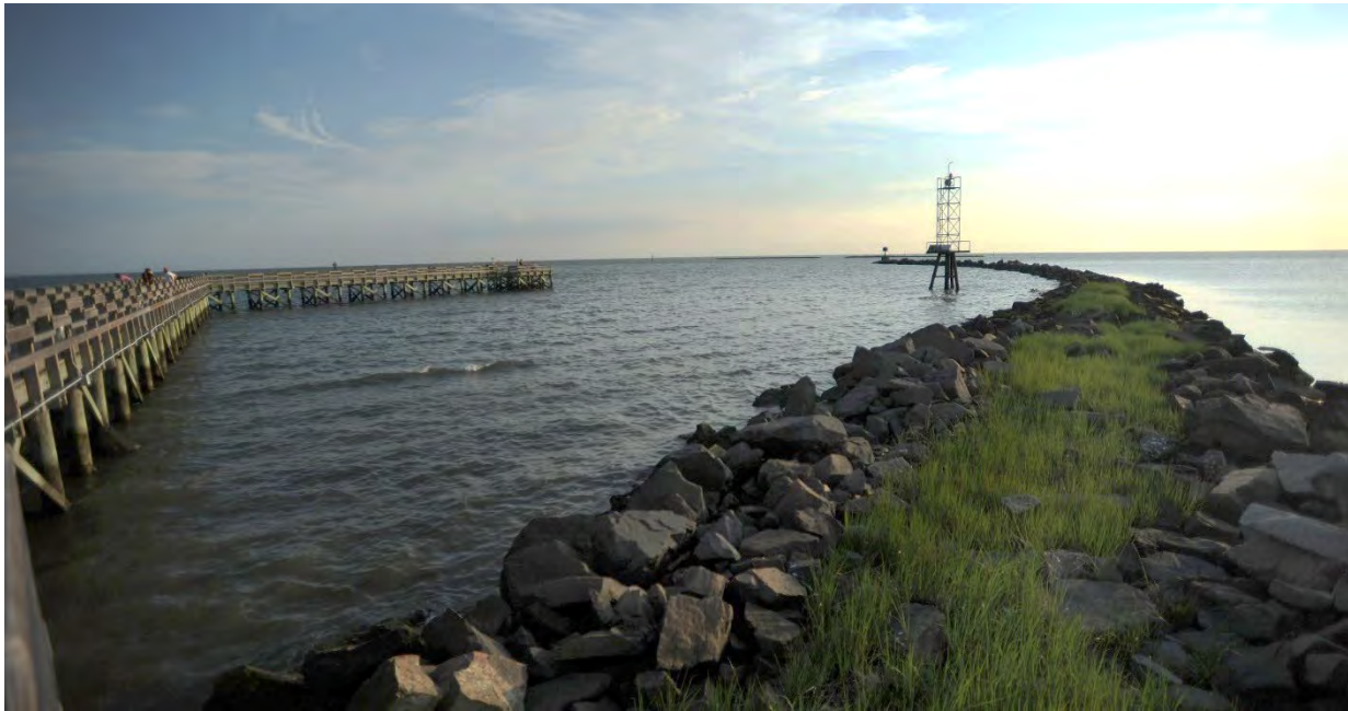
Figure 6: Jetty at Cape Charles Harbor. Photo Credit: Jay Diem, Eastern Shore News. Used with permission.
