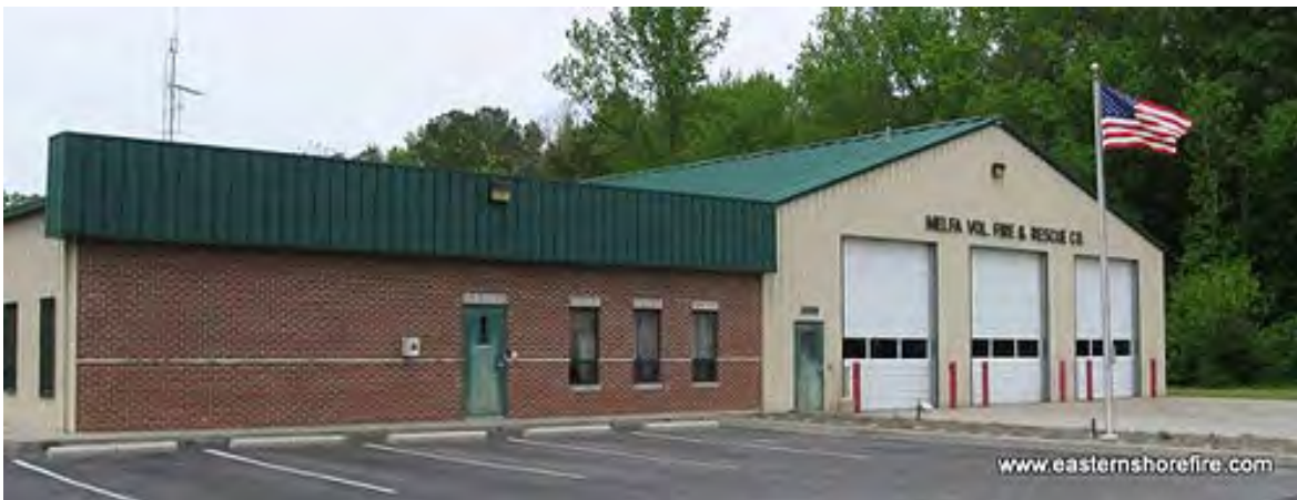
Figure 2 : Melfa Volunteer Fire and Rescue Company Station on Hatton Avenue
