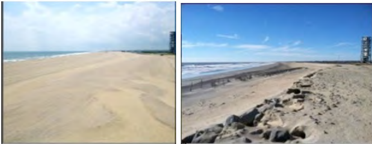
Figure 9: Beach Erosion at Wallops Flight Facility. Left: The completed beach nourishment project at WFF in August 2012. Right: The same stretch of beach is extensively eroded less than three months later, following Hurricane Sandy. Photo Credit: NASA
