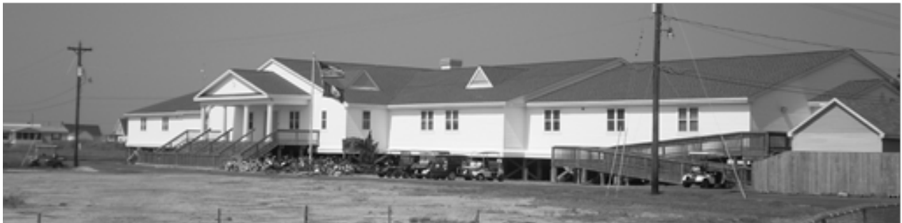
Figure 8: The Tangier Combined School was elevated in 2006 to mitigate flood damages. Photo by Curt Smith
